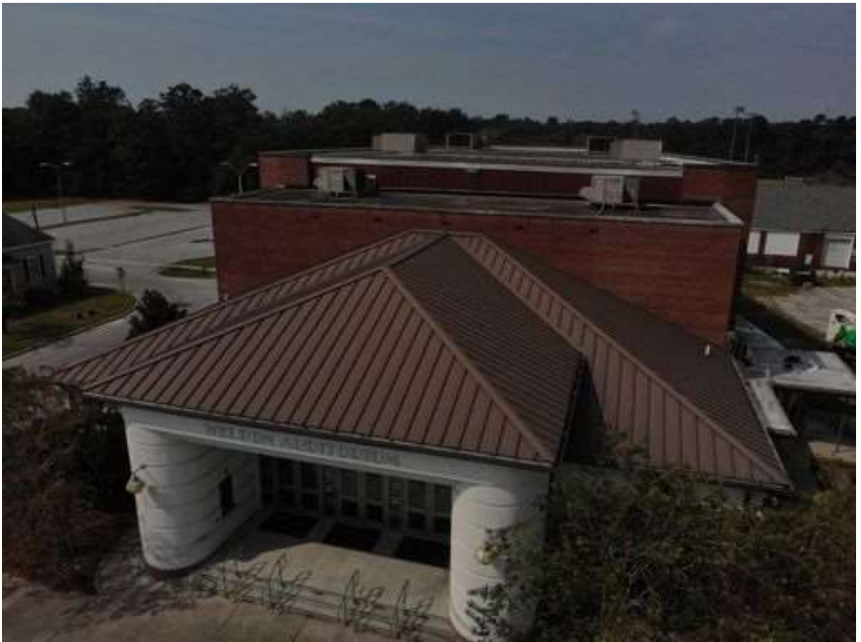
Photo 1: Front (East) Elevation of subject structure
