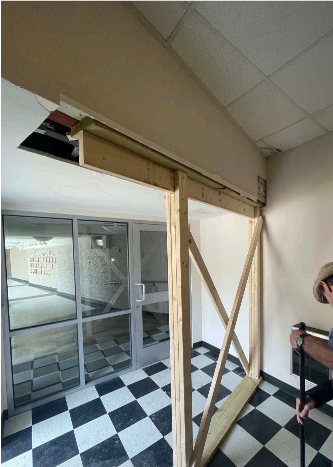
Figure 34: Weldon Auditorium: View of temporary stabilization.
