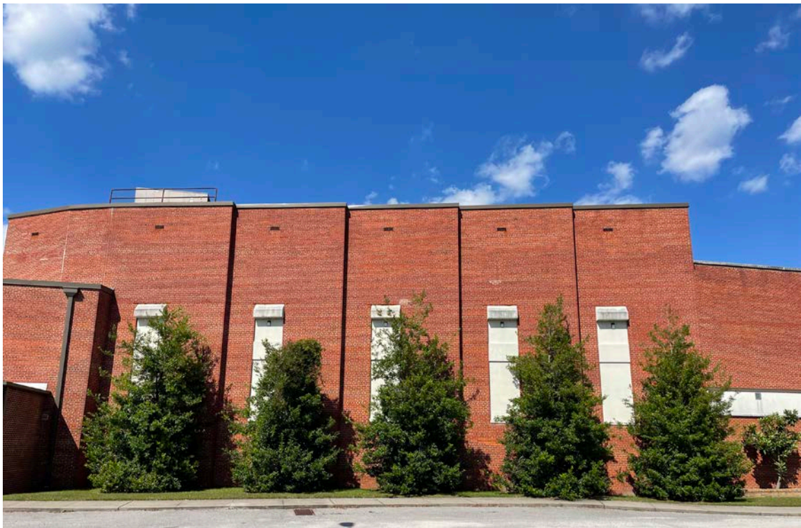
Figure 4: Weldon Auditorium: South Auditorium Elevation.
