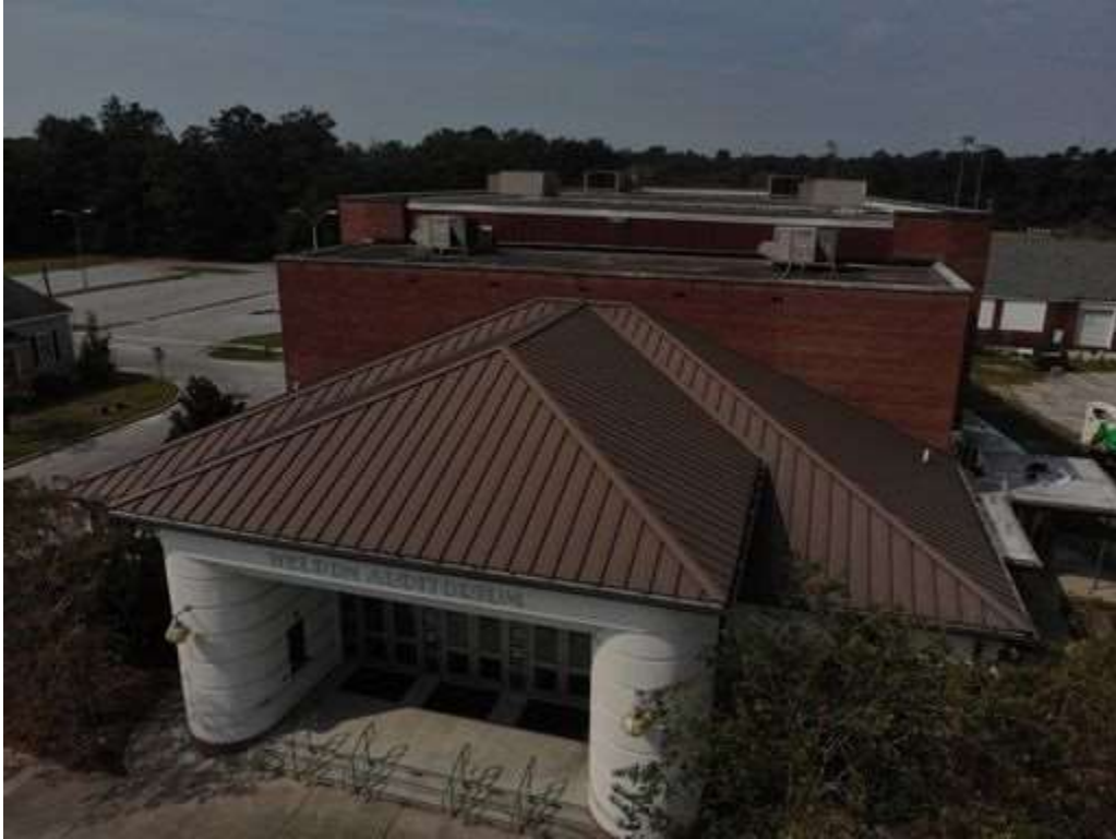
Photo 1: Front (East) Elevation of subject structure
