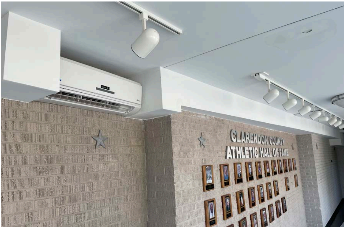
Figure 19: Weldon Auditorium: View of Ceiling Damage in Corridor Looking Southwest.
