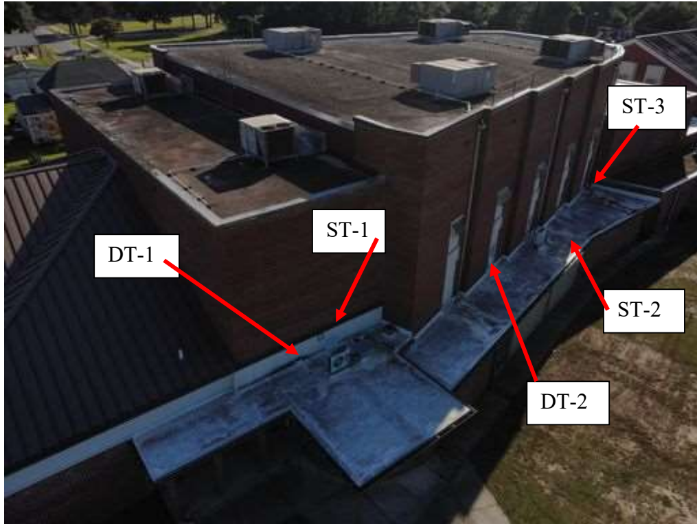
Photo 3: DT & ST locations at R8 & R7
