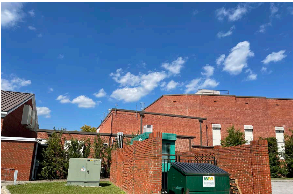
Figure 6: Weldon Auditorium: Southwest Corner.
