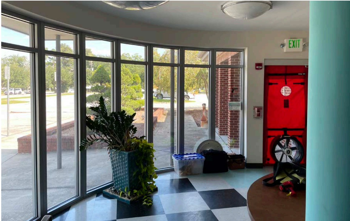
Figure 16: Weldon Auditorium: Art Walk Interior, Looking East.
