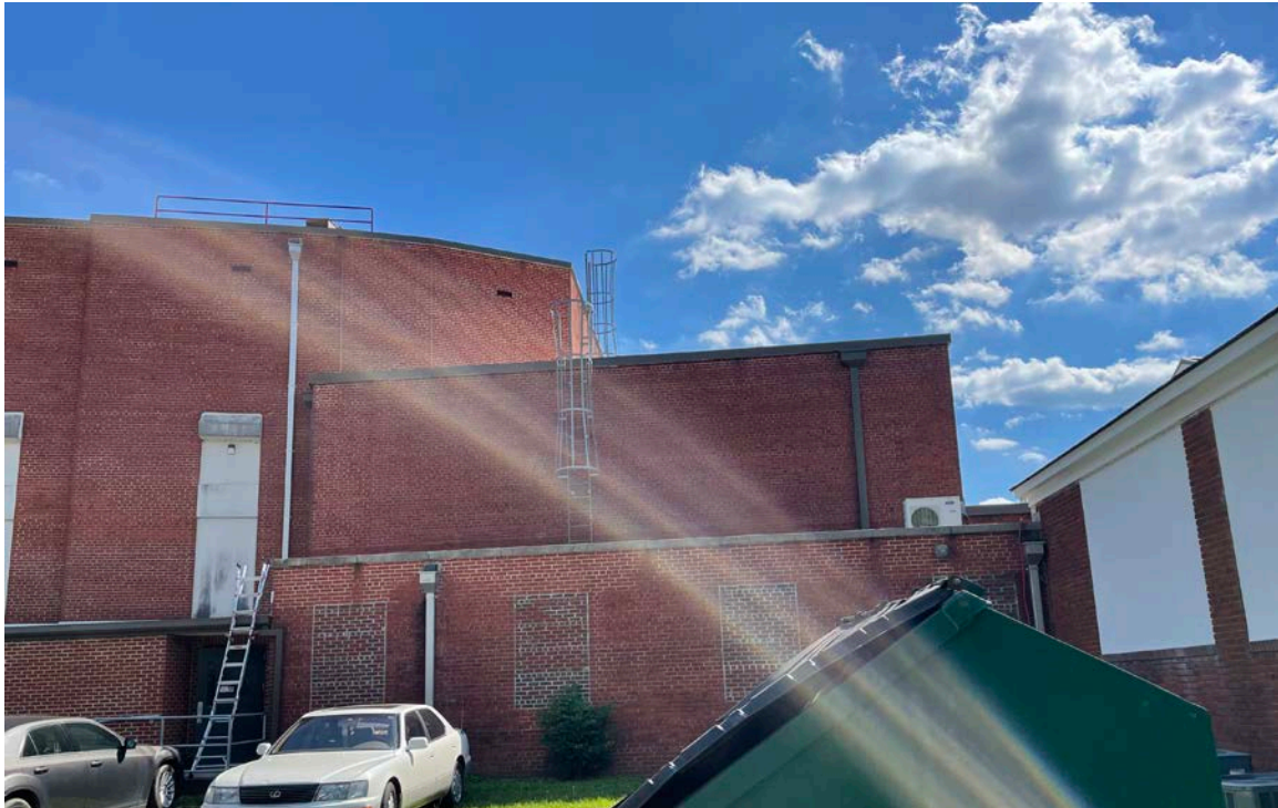
Figure 9: Weldon Auditorium: Northwest Corner.
