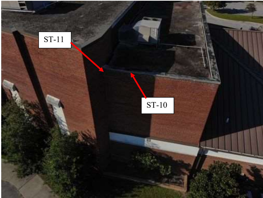
Photo 7: DT & ST locations at R2
