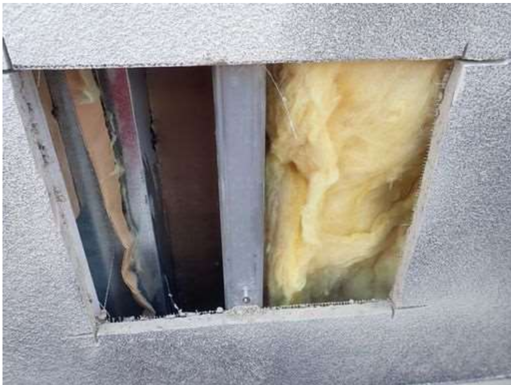
Photo 14: View of DT-2 at exterior cladding
