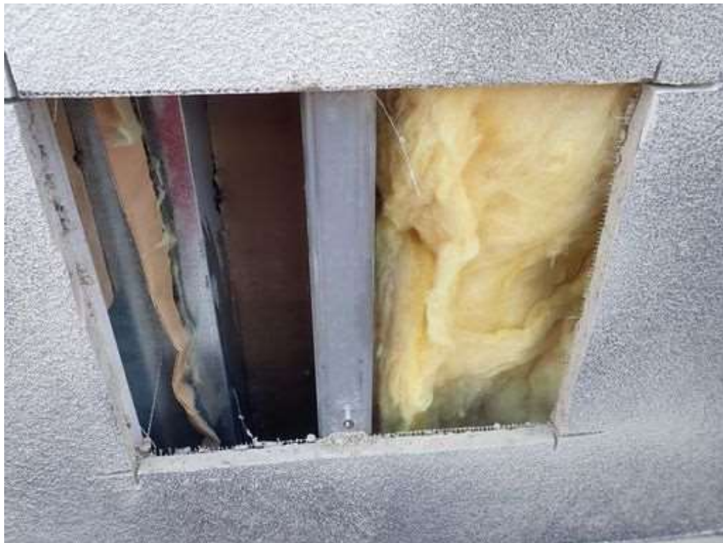
Photo 14: View of DT-2 at exterior cladding
