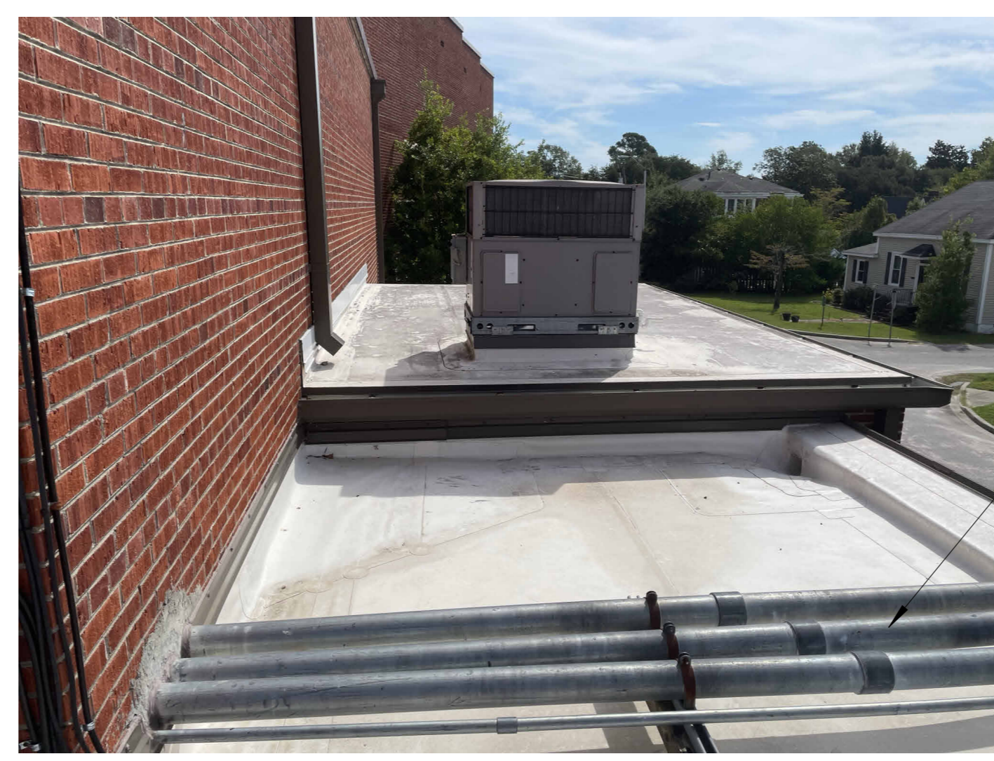
6 EXISTING ROOFING CONDITION AT ROOF G & D N.T.S.
