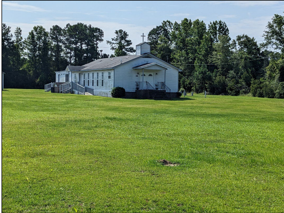
Figure 12. Community Deliverance Temple (0312), facing southeast.
