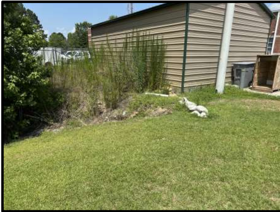
Photograph 17: Start of drainage feature toward the center of the subject property .
