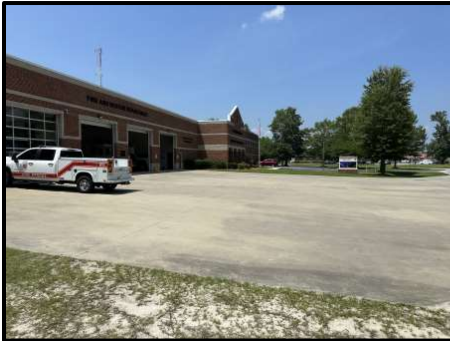
Photograph 2: Front entrances of Fire Station and Sheriff's Department.
