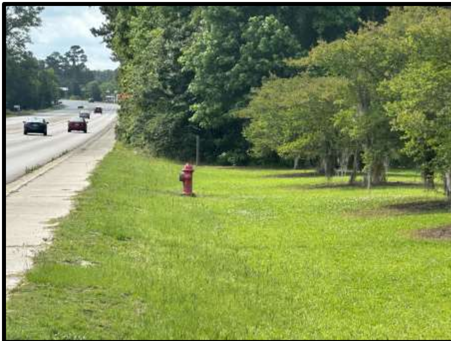
Photograph 4: Evidence of water infrastructure along northern boundary of subject property .
