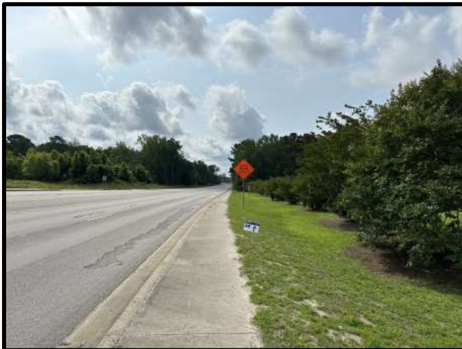
Photograph 2: Looking east along US Highway 378.
